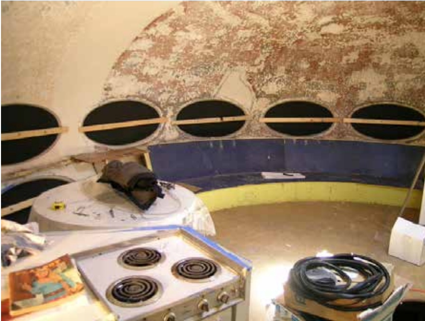
Figure 16 Installing the mock-up acrylic window in a mock-up fiberglass frame made by Mr. Donaldson at Planet Plastics, Corona, CA, May 22, 2003. Source: Donaldson.
