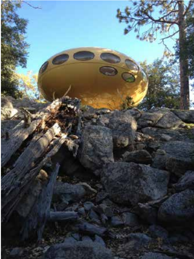
Photo 3 Exterior, Futuro on top of faux rock concrete footing, camera facing south
